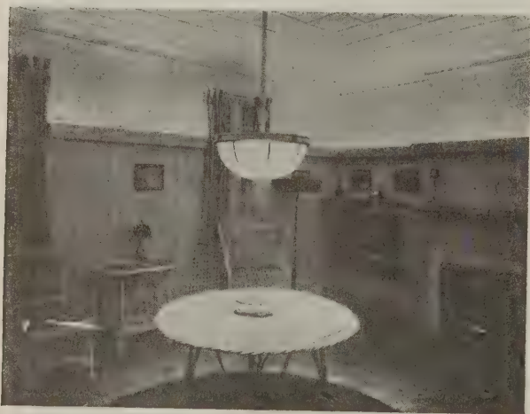
Fig. 5. A new type of dining room fixture which produces a combined effect of a semi-indirect unit and a powerful downward cone of light. This is an illustration of a demonstration room. The cove is emitting a low intensity of tinted light
